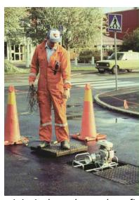
The mini winch can be made to fit different kind of man hole openings.
