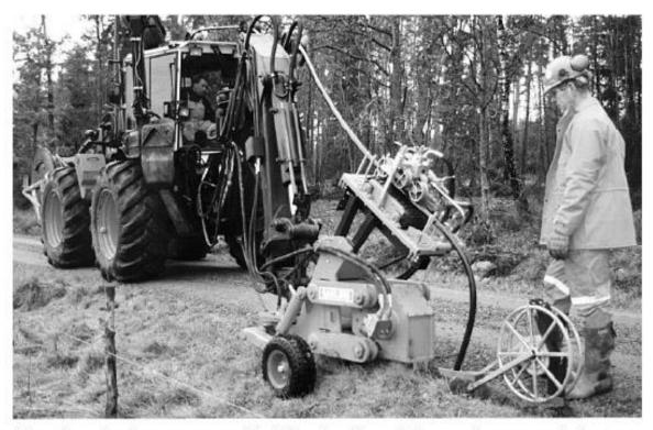
Vibration ploughs can cope with difficult soil conditions and are more lenient on the cable. Stones and small rocks are disposed of more easily and the furrow is filled again with fine grain material. The plough is fitted with a hydraulically operated support wheel to achieve the correct depth of trench. A turning attachment for lateral adjustment of the plough is provided. Vibration insulation between plough and machine.
